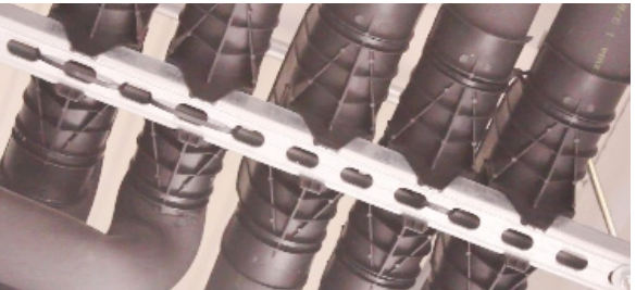
Figure 4-3. Piping support
