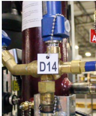
Figure 2-4 . Pressure Relief Valve Figure 2-5. Dual Manifold Pressure Relief Valve
