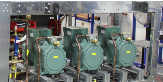
Figure 1-9. Medium temrerature compressor (MT)
