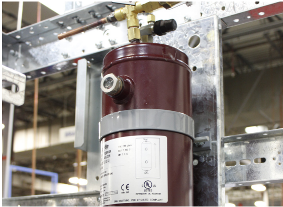
Figure 1-13. Oil reservoir
