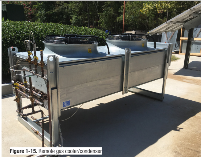
Figure 1-15. Remote gas cooler/condenser
