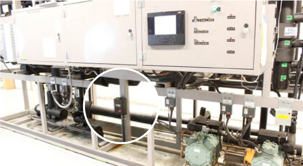
Figure 2-3. Example of a Leak Detection System
